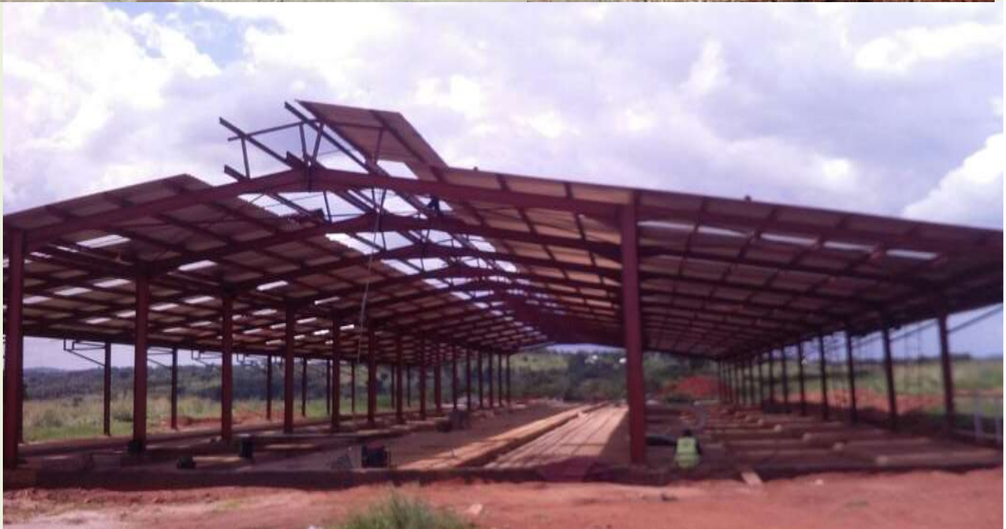
Fabrication and Erection of Cowshed portal frames for NARO, Namulonge, Uganda
